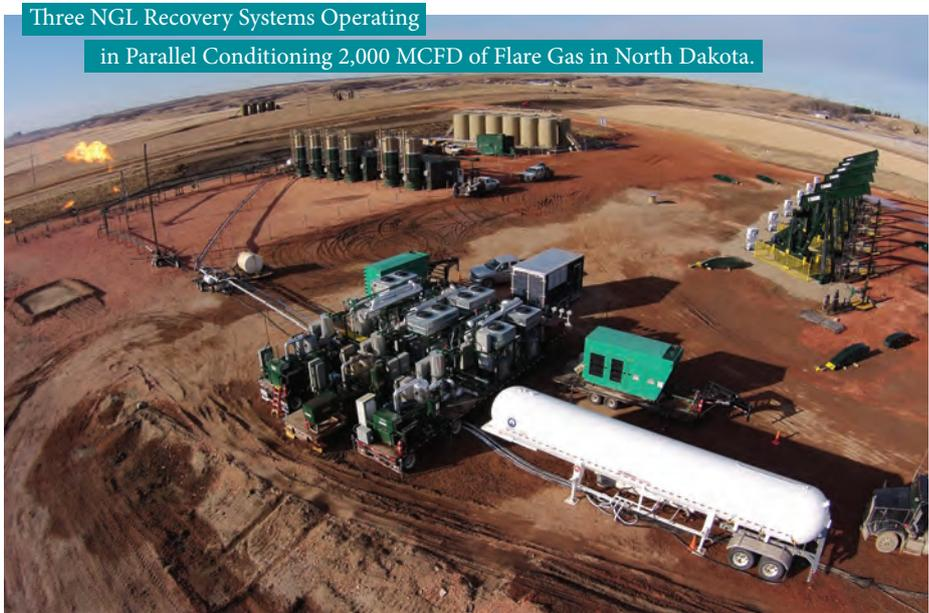
Three NGL Recovery Systems Operating in Parallel Conditioning 2,000 MCFD of Flare Gas in North Dakota.
